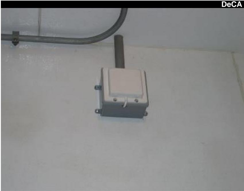
FIGURE 2: Each freezer and chill storage requires a 400-Series Cable with a RP-TNC plug on one end and a RP-TNC jack installed on the other end. The RP-TNC jack connector end of the 400-series cable will be installed into the 12" long by 3/4" NSF Plain End PVC conduit and terminate inside the 3/4" two gang Type FSE box installed in the freezer/chill storage. No more than 3" of the 400-Series Cable will be exposed inside the Type FSE box.
